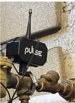
**Chad Sisco** of Energy & Engineering is leading an effort to install 20 Pulse Industrial meters strategically throughout campus. This is part of a pilot program to provide alerts via a system dashboard when a steam trap is starting to fail, and support energy-efficient operations.
