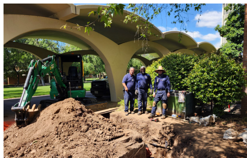
Irrigation replacement at Rivera Library (UCR/Mark Jones)
