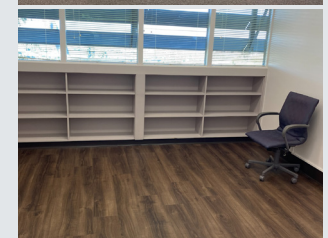
Space renovations (UCR/Dan Lerman)
